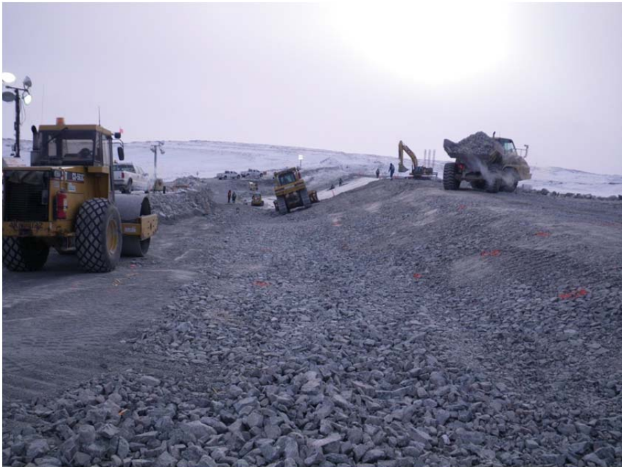
Photo 8: View of transition material placement. Photo looking south west along dam alignment.
