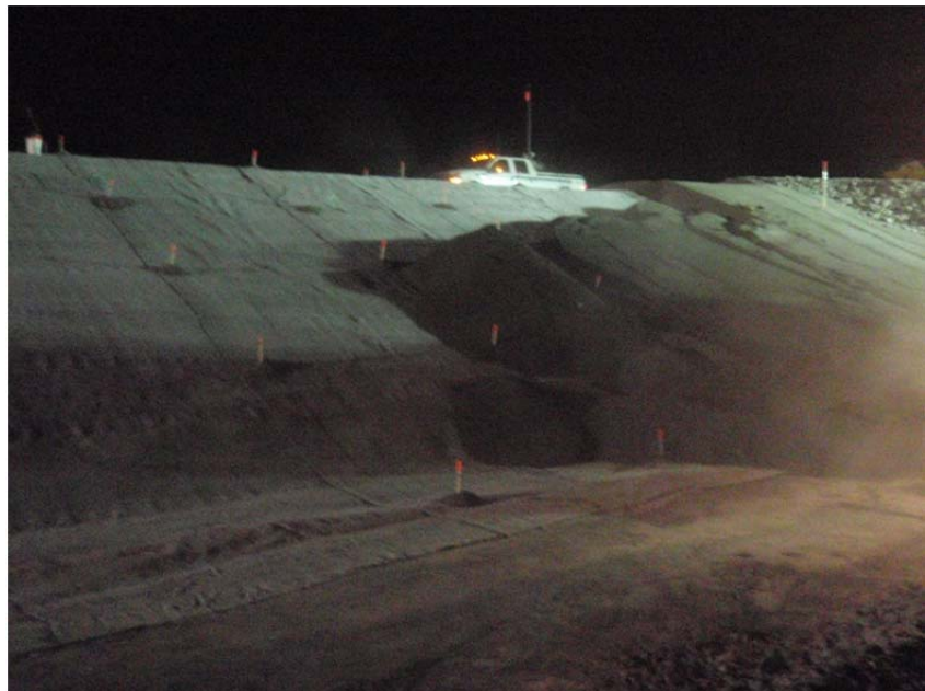
Photo 17: View of survey stakes placed for grade control for today's material placement.
