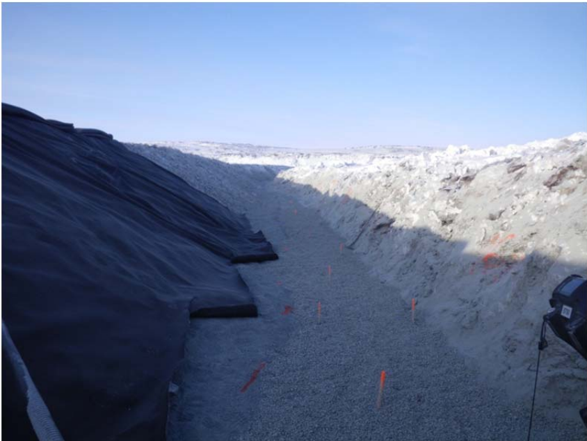
Photo 11: Compacted crush and bentonite at base of diversion berm key trench and lower geotextile. Photo looking west from station 1+60.
