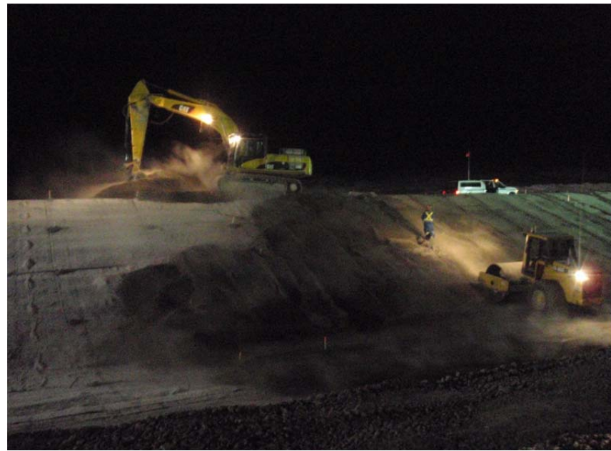
Photo 23: ~NWN view of Overliner material placement progress. Note that the survey stakes were attempted to be removed from a given area before the packer traveled over the Overliner material surface.
