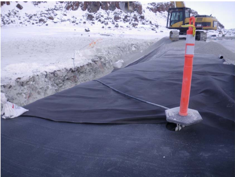
Photo 9: Diversion berm. Hole in liner at crest of berm for power cable near station 160.
