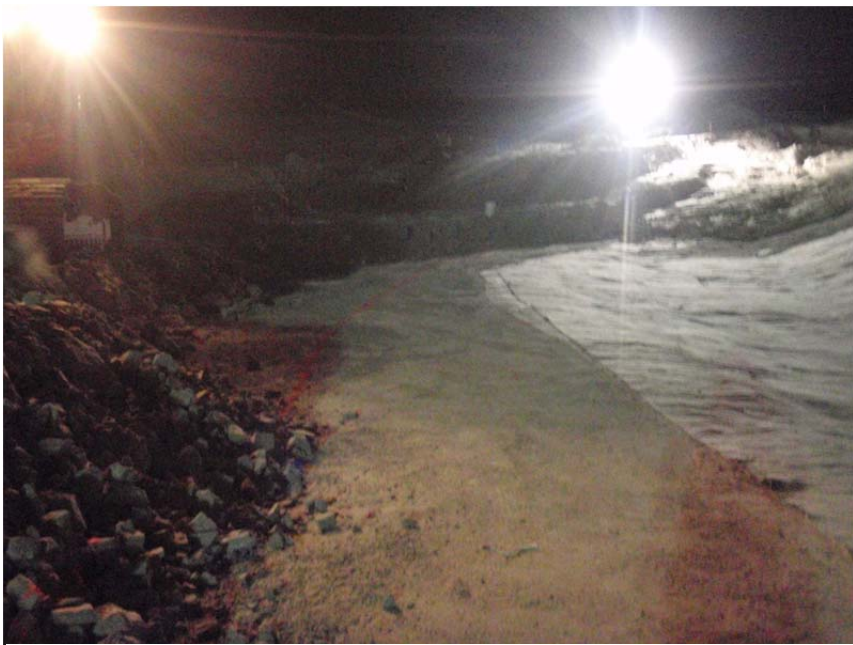
Photo 15: ~SSW view of the core fillet area. Note the orange liner denoted the x and y (easting and northing) extents of the design IFC fillet limits.
