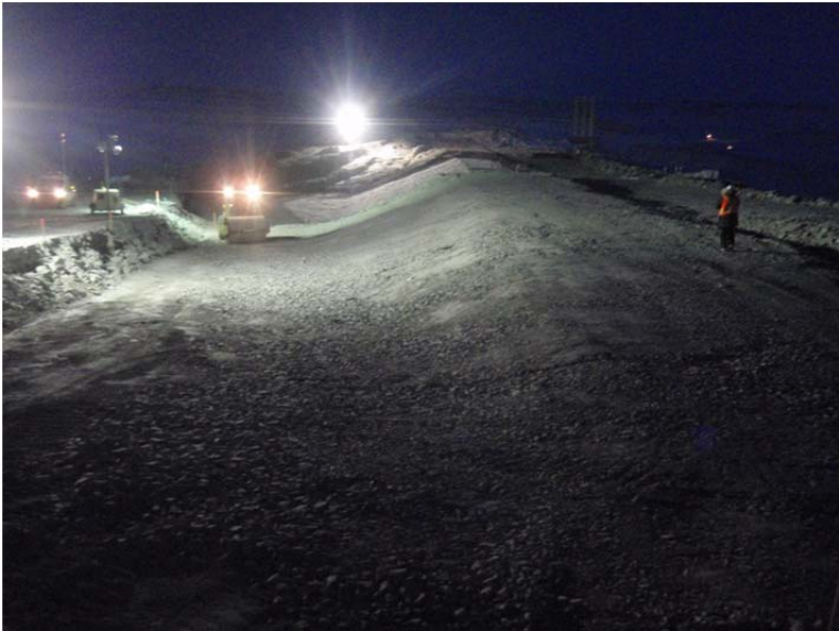
Photo 12: Placement of bentonite in base of diversion berm trench.
