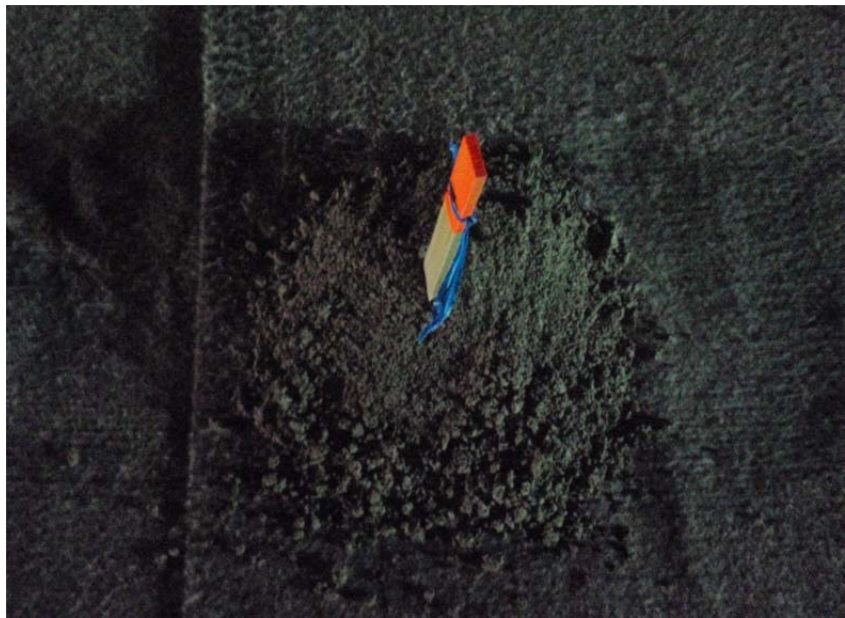
Photo 18: Note that the grade stakes were placed in some Overliner material after it had been hand shoveled onto the area around the GCL seams. Stakes were only placed around the seams as this area has a little more cushioning in case a stake was accidentally pushed through the Overliner fill towards the GCL surface.
