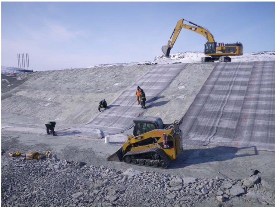
Photo 7: Placement of GCL along the slope near station 1+05.
