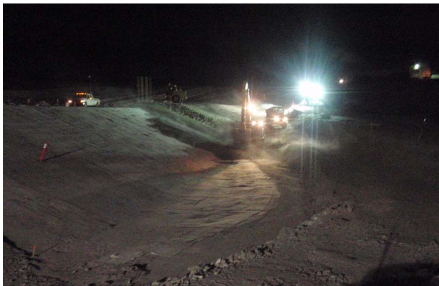
Photo 22: ~ NNE view down the upstream dam core slope towards Overliner placement activities. Taken from around 0+70 on the upstream shell corner area.
