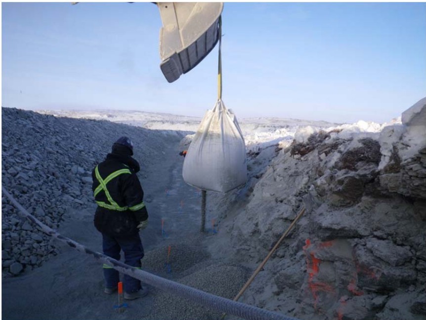
Photo 12: Placement of bentonite in base of diversion berm trench.
