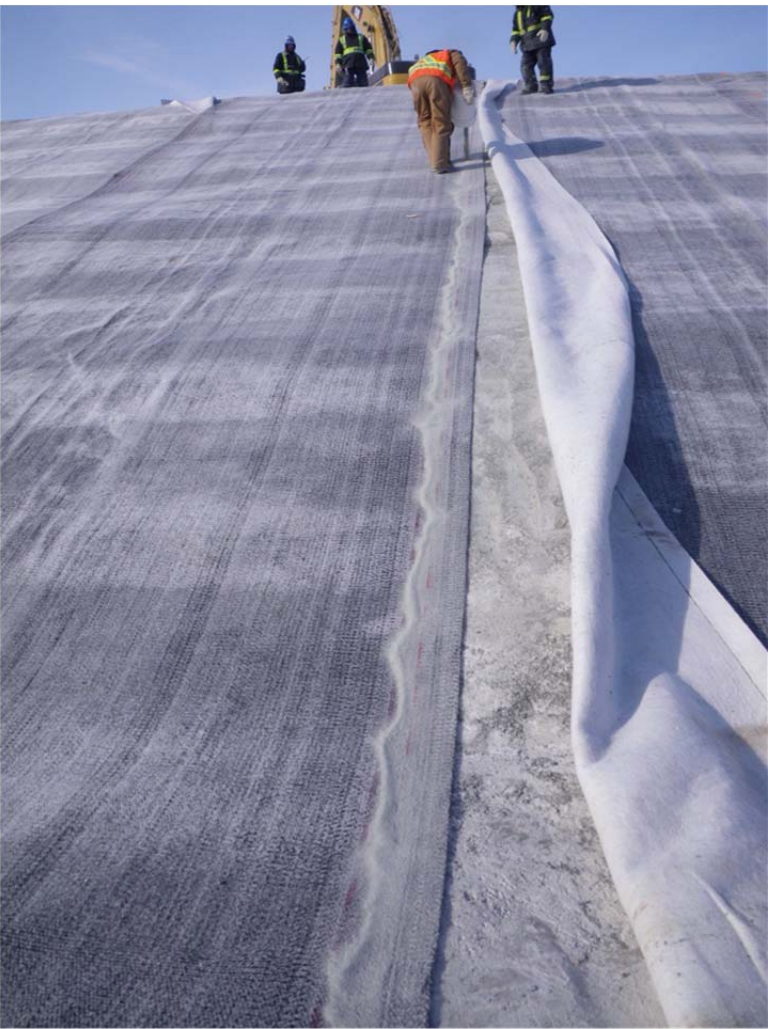
Photo 4 (above): Bentonite being placed along overlap between sections of GCL.
