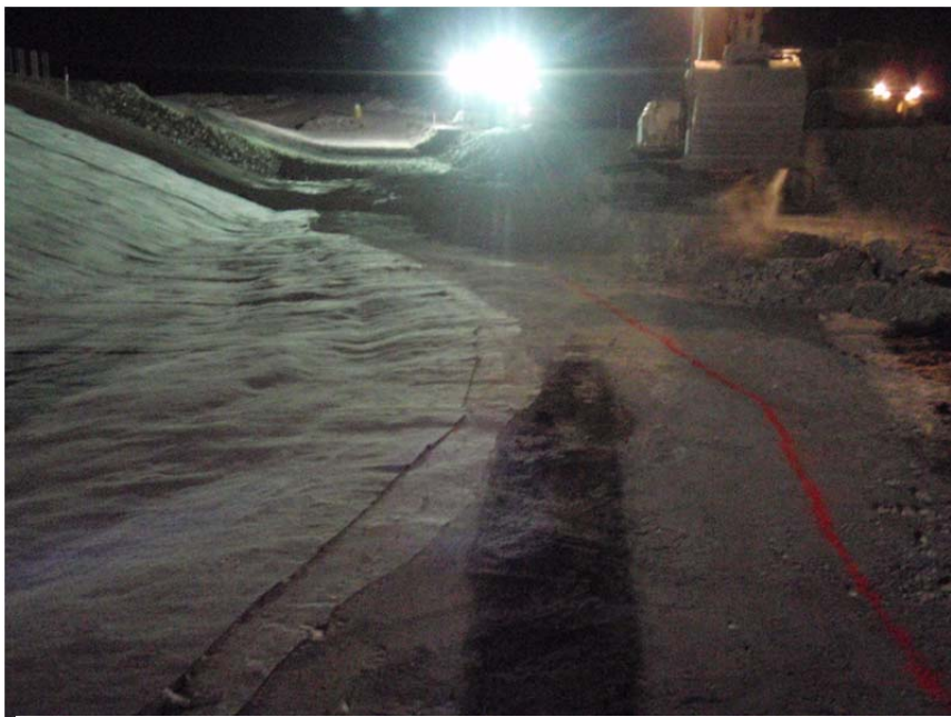
Photo 16: ~NNE view of the core fillet area. Note the orange liner denoted the x and y (easting and northing) extents of the design IFC fillet limits.
