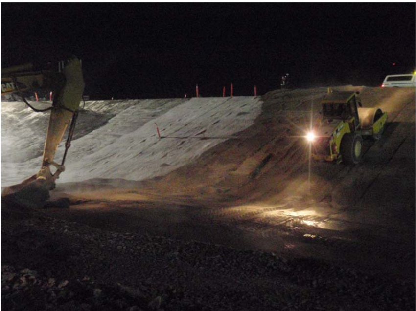
Photo 24: ~ NE view of the end of today's Overliner placement. Note ~15m of CL still remained exposed at the end of the shift.
